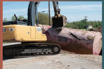
The underground gas tanks were excavated and the gas pumps were dismantled at the former One Stop in Kaw City.
